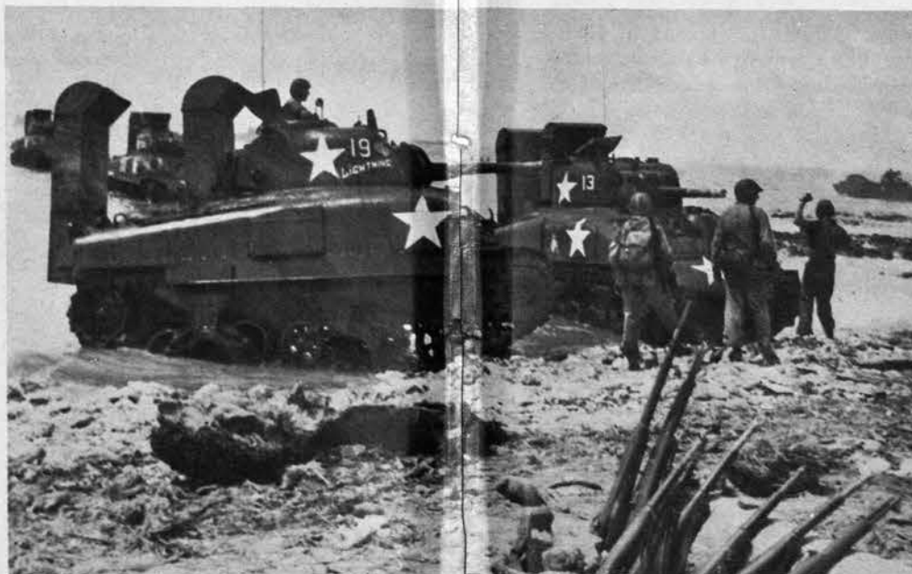
Invading Sherman tanks now hitting the beaches are appearing with a new silhouette. Tall, removable periscope-like
